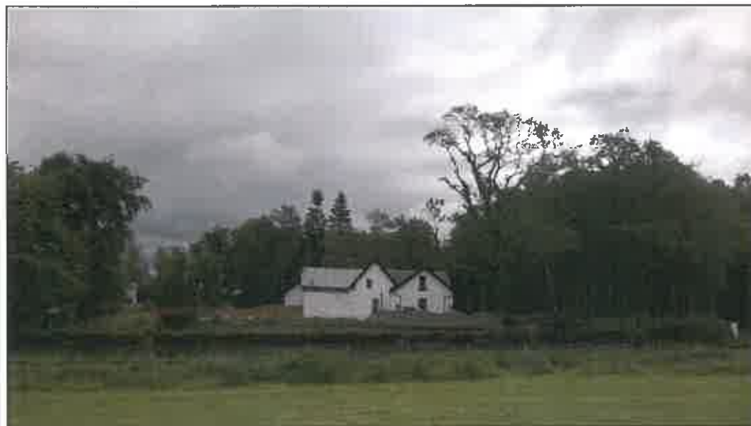
Fig 2: Application Site from the west
